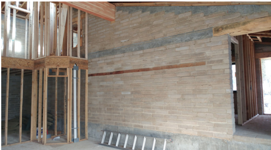
Interior walls under construction.
