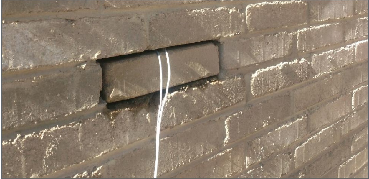
Image16: A CEB block equipped with the embedded sensors, as installed in a CEB wall in the Castle Rock project.
